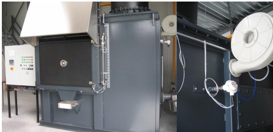
Example of Jongtech incinerator with an Econox HT probe
